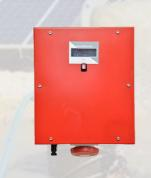
The controller is an electric device that matches the power output from the solar Structure to the pump motor and regulates the Operation of the pump according to the input energy from solar array.
